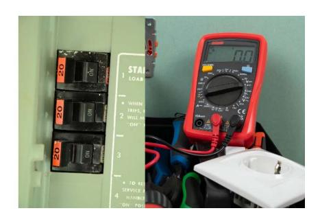
One of the crucial aspects of testing and inspection is identifying the presence of FPE Panel Stab-Lok circuit breakers. These breakers have been found to have significant design flaws, which may result in breakers failing to trip when needed. This can lead to overheating, electrical fires, or even electrocution hazards.
